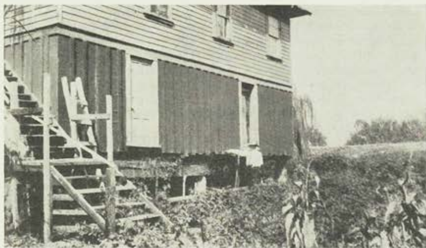
Fig. 4: House on Lower Jones Tract built upon piling. The peat soil surrounding this house has subsided more than 4 feet in about 20 years.
